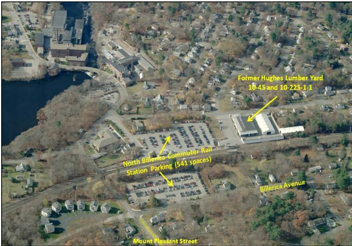
Image 7: Former Hughes Lumber Yard near the intersection of Billerica Avenue and Mount Pleasant Street
