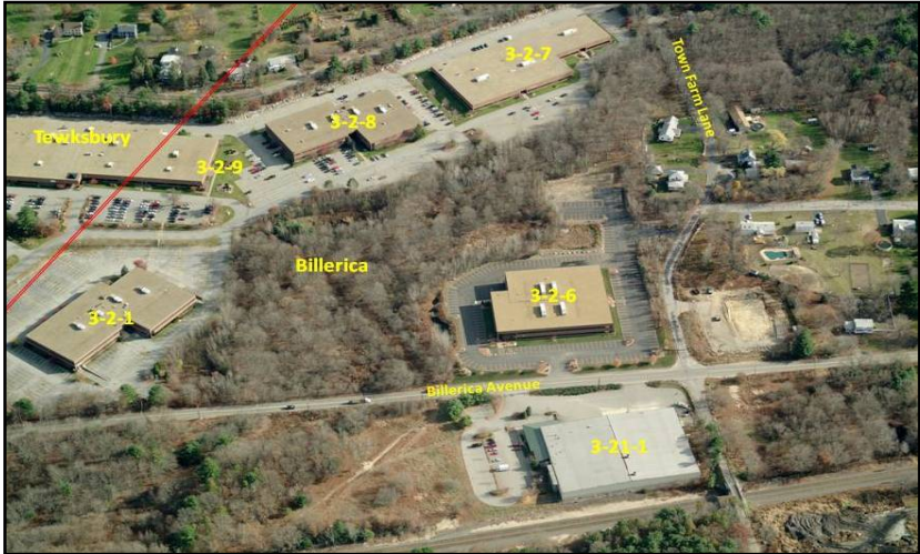
Image 8: Several of the commercial office buildings are fully vacant as you can see at parcel 3-2-6 and 3-2-1.
