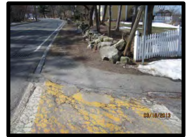
Photo 28: Depot Street south of Beaver Dam Drive.
