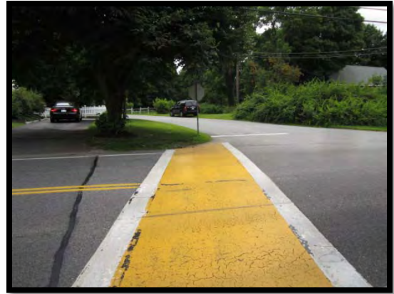
Photo 16: Crosswalk on Depot St by Fisher Way.
