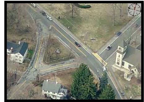
Photo 10: Intersection of Boston Rd./ Hildreth St. and Lincoln St.
