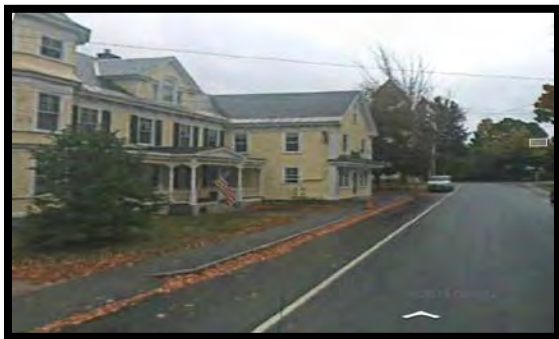
Photo 14: Sidewalk on Lincoln St.
