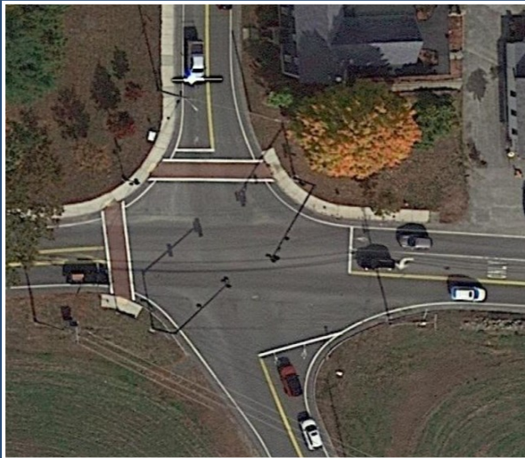
Above: East Street at Livingston Street in Tewksbury with improvements programmed in the 2011 TIP.
