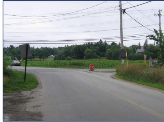
Photo 3: Livingston Street Southbound Approach to East Street before Improvements (2008)
