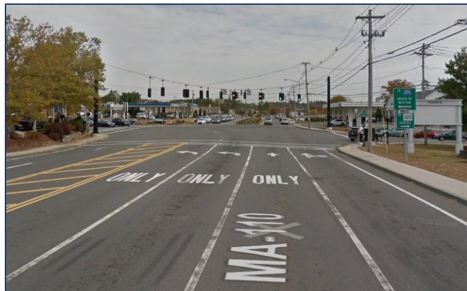
Photo 7: Littleton Road Eastbound Approach to Boston Road after Improvements (2018)
