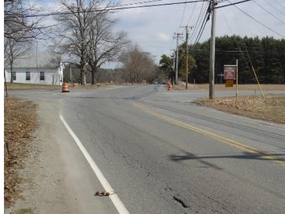
Photo 1: East Street Eastbound Approach to Livingston Street (Pre Construction)
