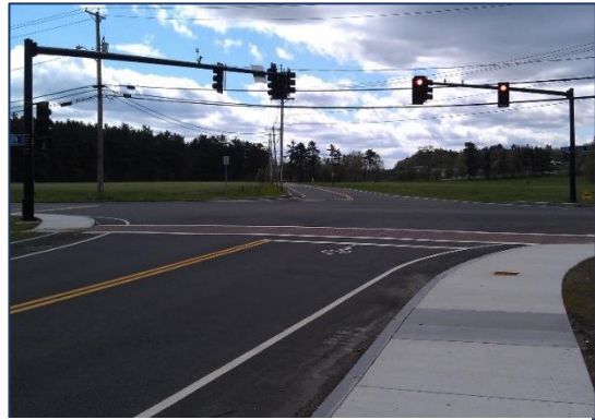
Photo 4: Livingston Street Southbound Approach to East Street after Improvements (2012)
