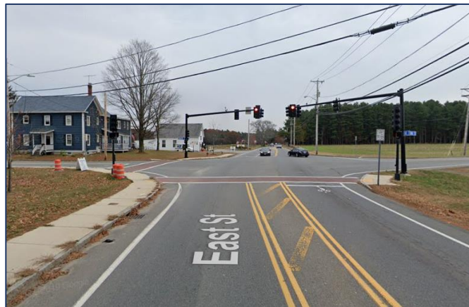
Photo 2: East Street Eastbound Approach to Livingston Street Post Construction (2019)
