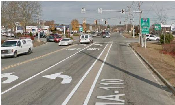
Photo 19: Minot's Corner Before improvements (2012) Eastbound Route 110 approach (Source: Google Maps)
