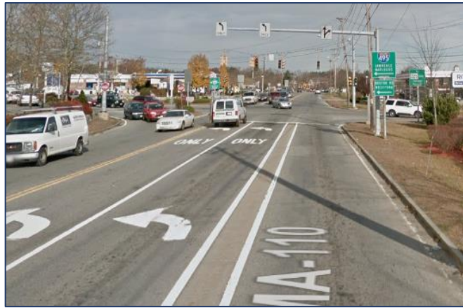
Photo 6: Littleton Road Eastbound Approach to Boston Road before Improvements (2012)
