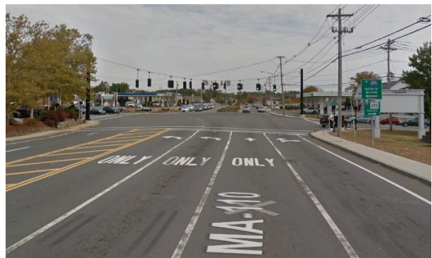
Photo 20: Minot's Corner After improvements (2018) Eastbound Route 110 approach (Source: Google Maps)
