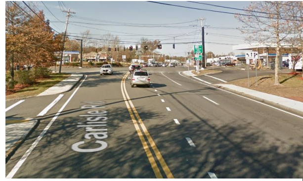
Photo 24: Minot's Corner After improvements (2018) Northbound Carlisle Road approach (Source: Google Maps)
