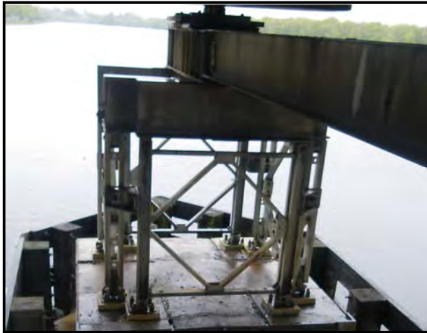
Figure 2-20 Typical Acrow Panel Tower
