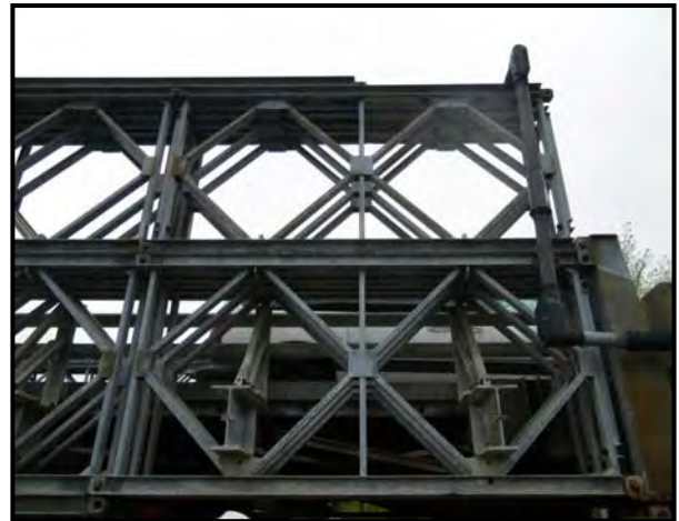
Figure 2-18 Beginning of Lamination/Section Loss
