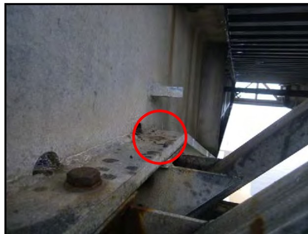
Figure 2-19 Sheared Bolt at the End of a Trussom
