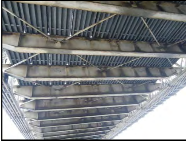
Figure 2-17 Typical Failure in Galvanized Coating
