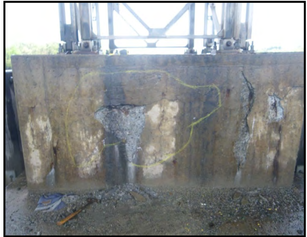
Figure 2-21 West Concrete Pedestal at Pier 3
