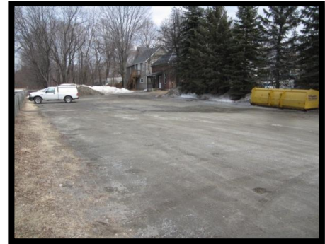
PHOTO 21: NRRT PARKING LOT OFF GROTON ST
