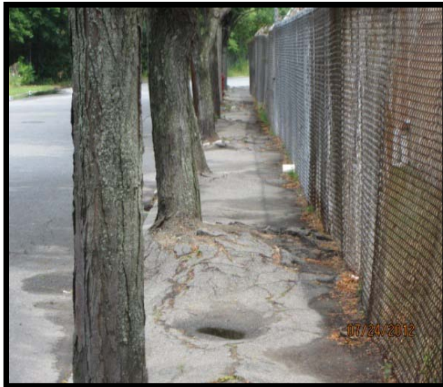
Photo 15: tree roots pushing through the sidewalk on Meadowcroft St.
