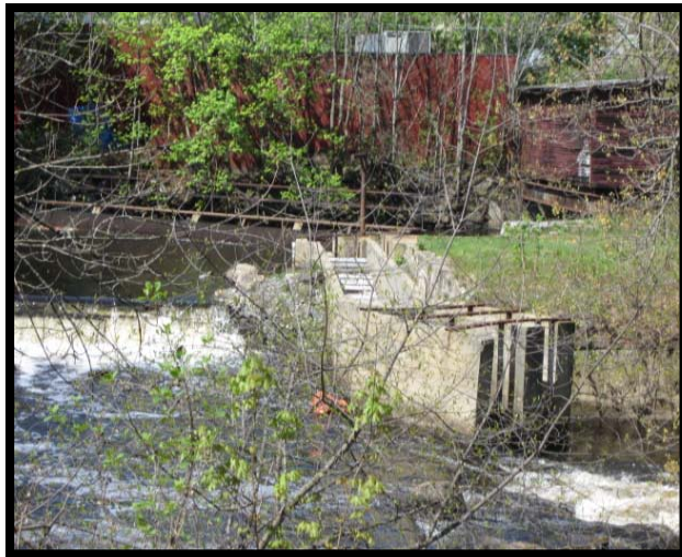
Photo 3: Dam at the Concord River Greenway
