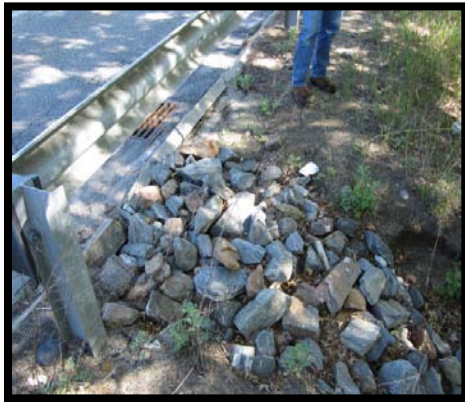
Photo 7: Drainage structure on the Lowell Connector.
