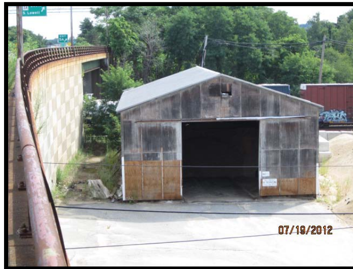
Photo 6: MassDOT owned salt shed on Howard St.
