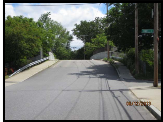
Photo 16: Bridge over railroad tracks on Lundberg St.
