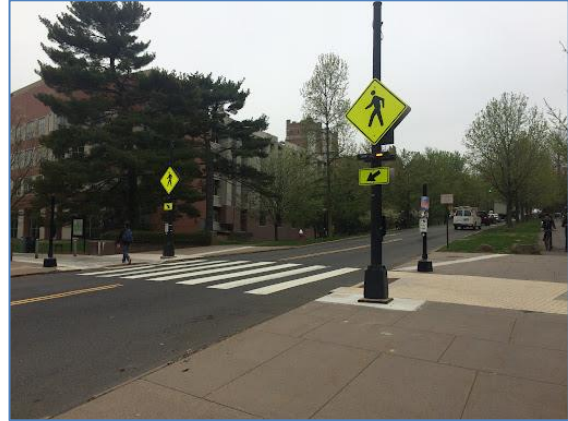
Photo 5: Example of a Rectangular Rapid Reflecting Beacon at a Crosswalk
