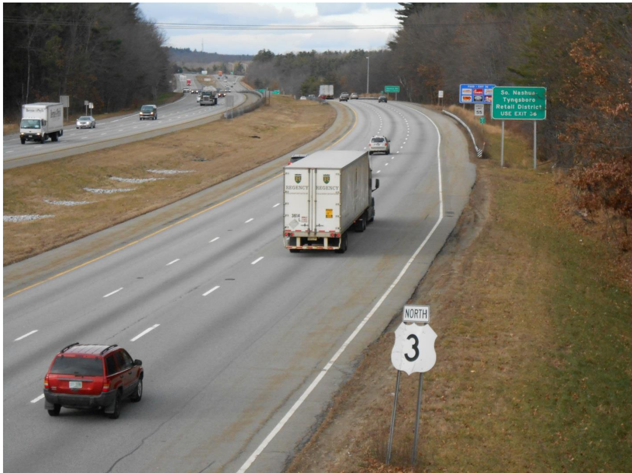
U.S. Route 3 looking north toward Exit 36 in Tyngsborough. (Credit: NRPC)
