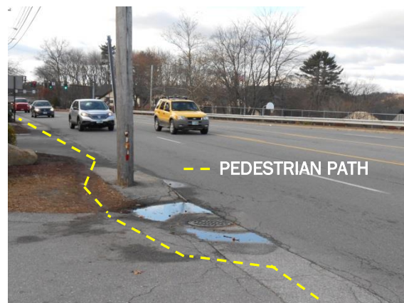
The placement of this utility pole on Spit Brook Road impedes pedestrian flow and a poorly sited storm drain causes water to accumulate in the pedestrian path.
