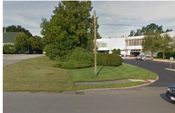
This sidewalk in front of a furniture store on Daniel Webster Highway terminates abruptly approximately 300 feet north of Exit 36.
