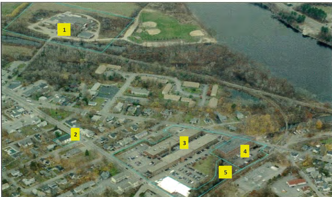
Aerial imagery of Vinal Square and the North Chelmsford Mill District. (Source: Pictometry International, 2008)
