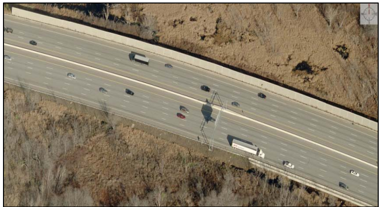
Picture 3 Route 3 Bottleneck North of Route 110 in Chelmsford
