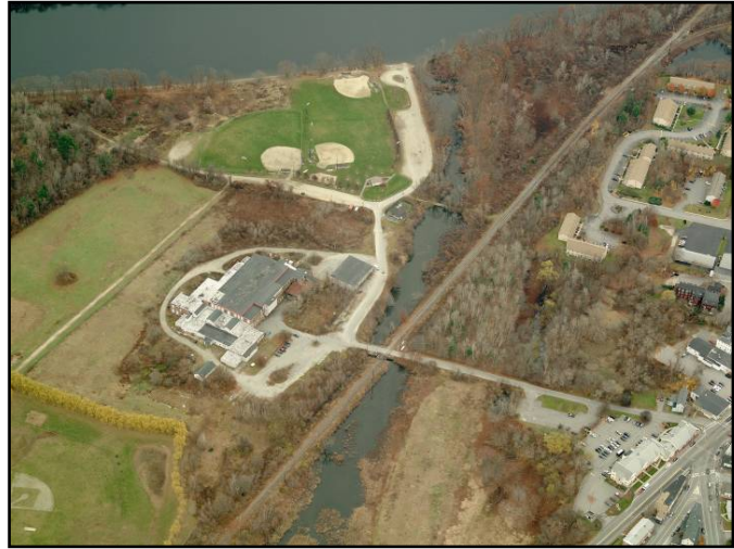
Potential redevelopment site for a new MBTA commuter rail station in Vinal Square. (Source: Pictometry International, 2008)
